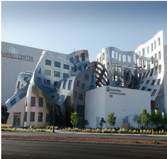
Fig. 1. Cleveland Clinic Lou Ruvo Centre for Brian Health. 2005-2010. Las Vegas, Nevada, USA. Architect, Frank Gehry
