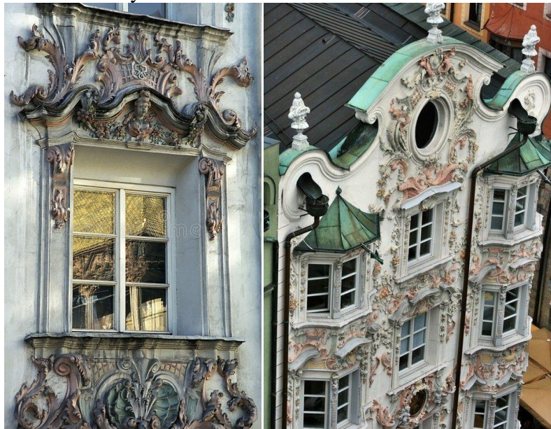
Picture 1. Framing for windows
